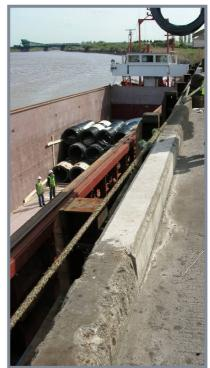
were to provide new fendering, execute specialist concrete repairs to the damaged concrete and to strengthen the buckled jetty pile.
